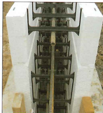
T wo layers of 2 1/2-inch-thick Styrofoam are held together by polypropylene ties with rebar guides and furring strips to attach drywall or exterior finish. Poured concrete sets up eight inches thick, with rebar at 16-inch intervals. The Styrofoam remains as insulation.
