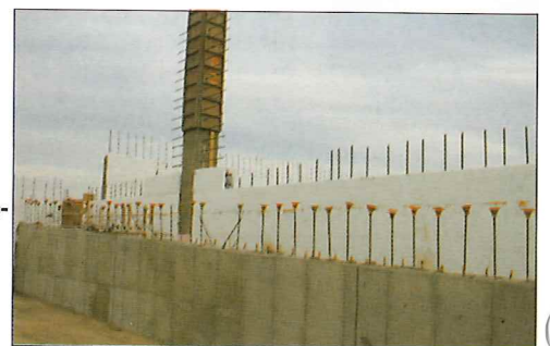
T wo layers of 2 1/2-inch-thick Styrofoam are held together by polypropylene ties with rebar guides and furring strips to attach drywall or exterior finish. Poured concrete sets up eight inches thick, with rebar at 16-inch intervals. The Styrofoam remains as insulation.
