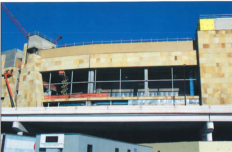
When finished, the crew from Seal Treat, Inc. will have completed approximately 17 miles of caulking throughout the entire precast of the new Twins Ballpark. Photo by Richard Kentzelman.
