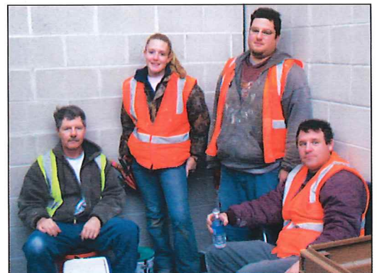
Masonry caulkers Dan Dahedl, Renee Ritter, Matt Tix, and John Salmon of Carciofini Company take a break from the cold, brutal temperatures of December while working at the new Twins Ballpark. Photo by Richard Kentzelman.
