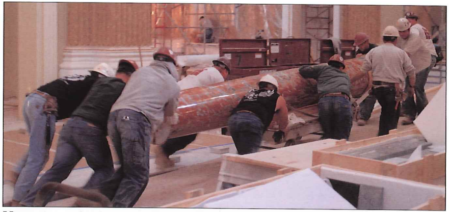
Manpower, wheels and pulleys built Medieval cathedrals, and they've been used here. Every available workman put his back into pushing the 7,000-pound marble column up a 40-foot ramp to be raised into place. The column rode on a cart whose rubber wheels protected the marble floor.
