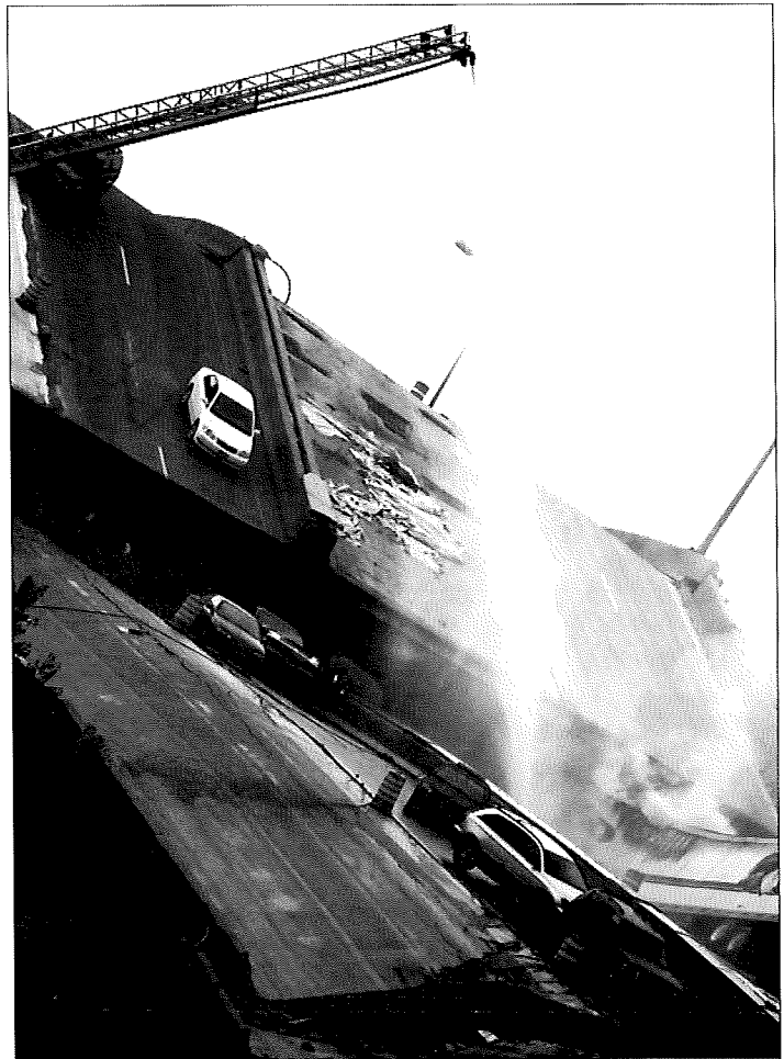
In this photo taken soon after the collapse, Babineau's truck, its lights still on, is seen wedged into the bridge wreckage. Just above is the white car that, to his amazement, never fell on him.
