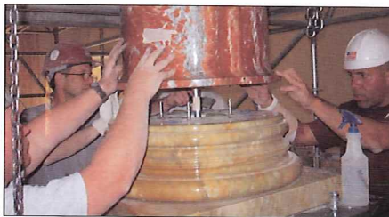
Manpower, wheels and pulleys built Medieval cathedrals, and they've been used here. Every available workman put his back into pushing the 7,000-pound marble column up a 40-foot ramp to be raised into place. The column rode on a cart whose rubber wheels protected the marble floor.
