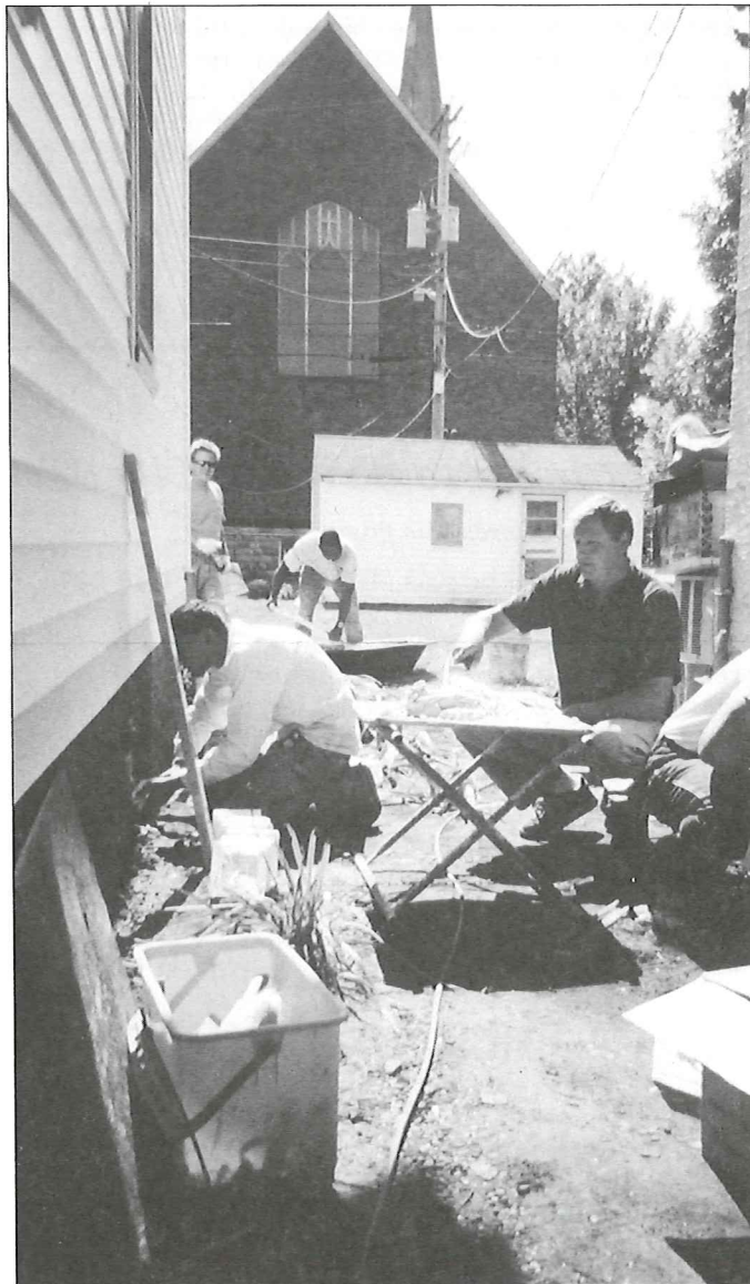
Peter Damyán of Minnetonka turns mortar with a trowel.
